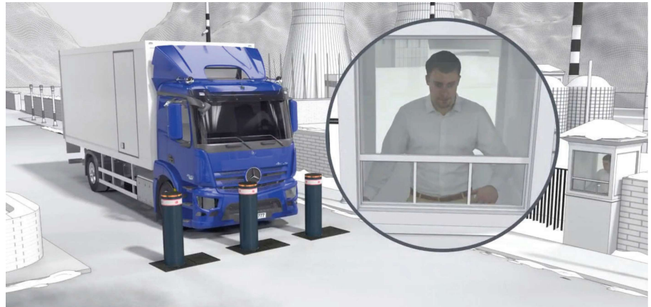
A security guard is able to use an emergency fast operation setting to activate bollards
