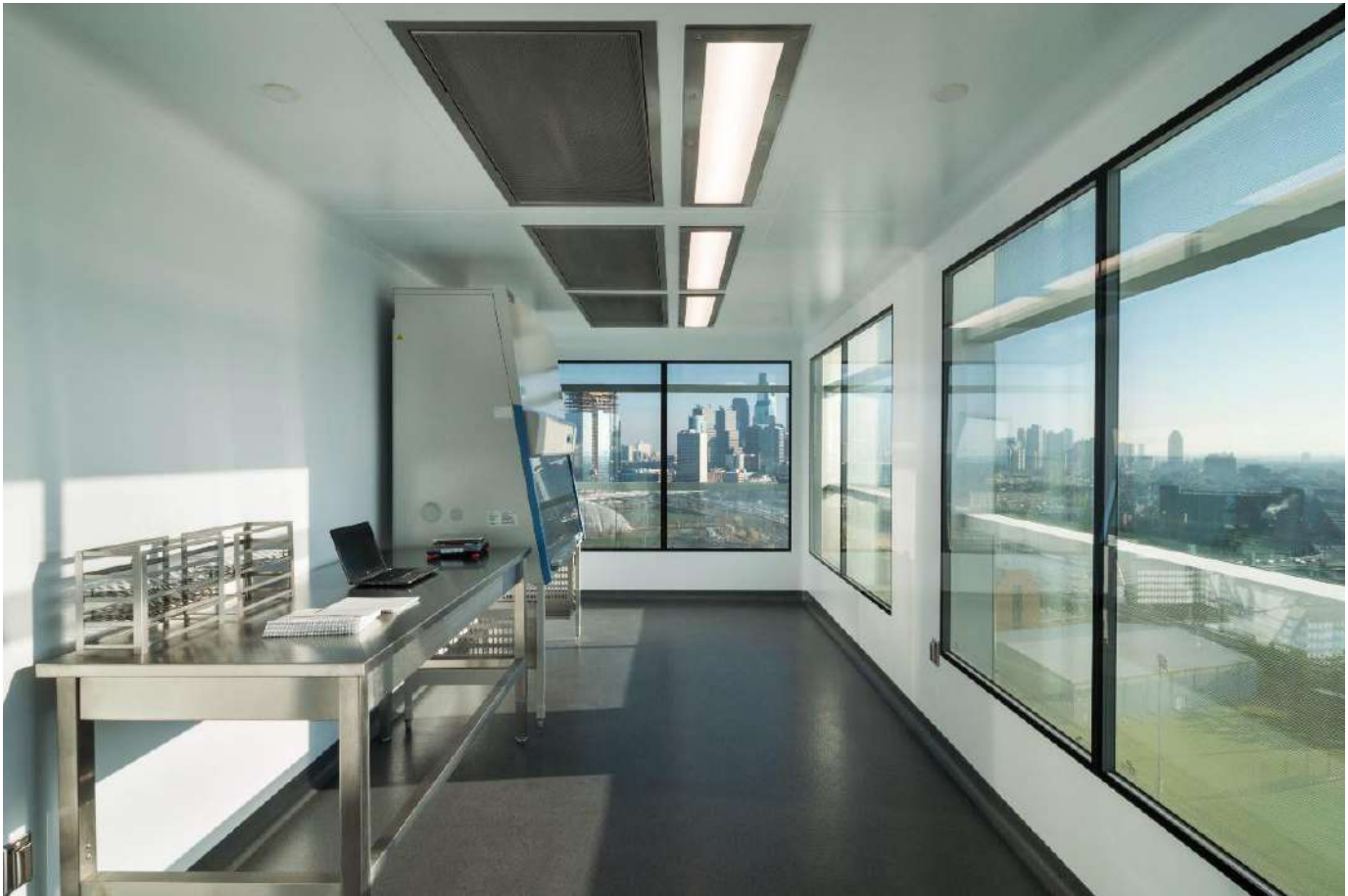
Shown here is a cleanroom facility responsible for a CAR-T treatment that was located on the 9th floor of a 16-story building on an urban hospital campus. Presenting challenging project logistics, the existing space compressed the cleanroom facility both horizontally and vertically due to extremely low floor-to-floor heights. Hugging the all-glass exterior of the skyscraper's custom envelope, the cleanroom facility's modular technology allowed it to wrap around the process and protect patient material while maintaining the views of the surrounding cityscape.
